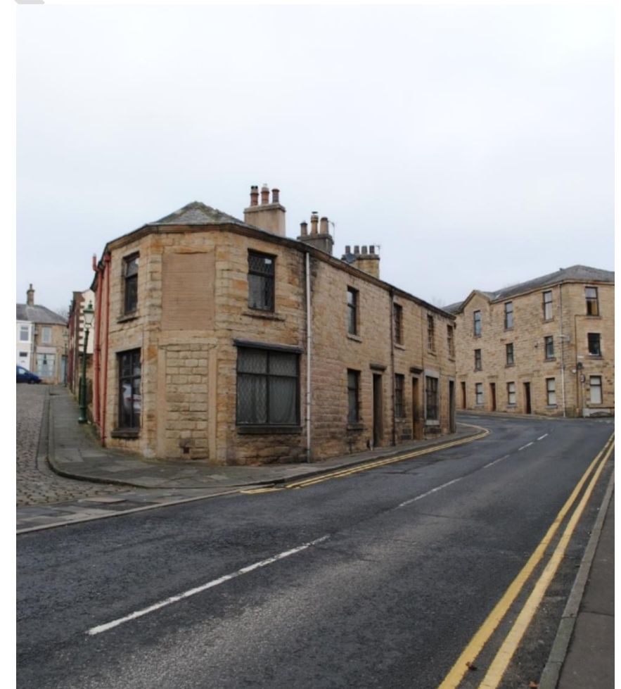
Figure 22 View of Moor Lane from the corner of Moor Lane and Burnley Road
