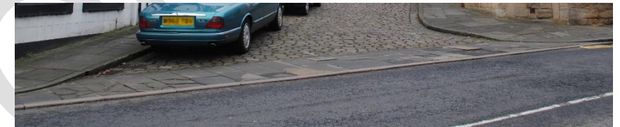
Figure 26 3 different surfaces at the junction between Moor Lane and Gawthorpe Street
