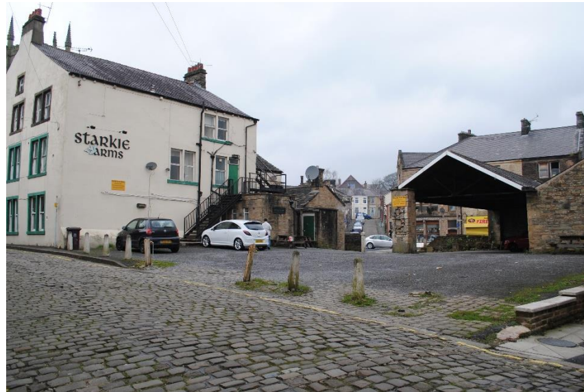
Figure 23 Car Park to rear of the Starkie Arms
