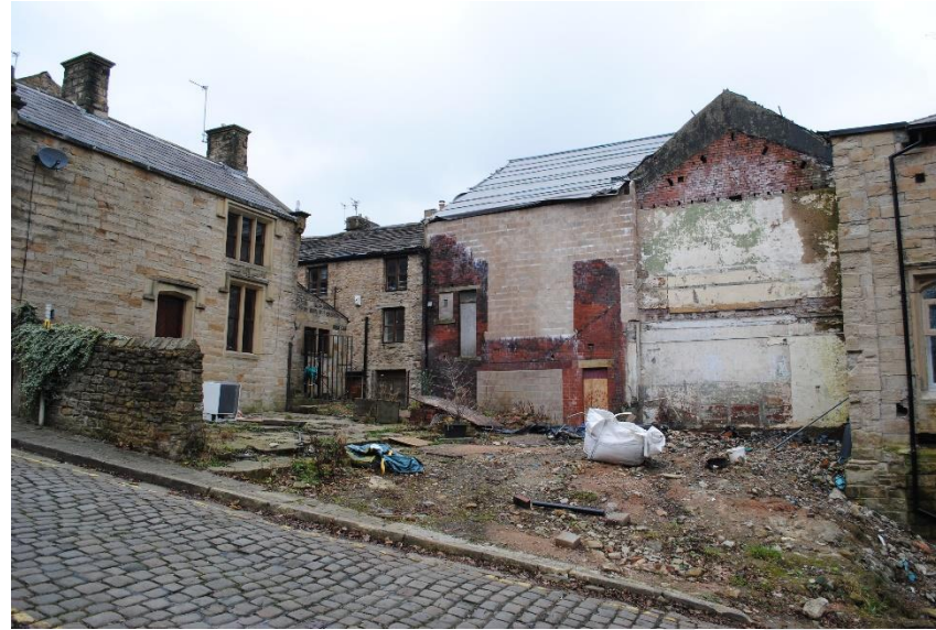
Figure 32 Gap site having a negative impact on Mill Street
