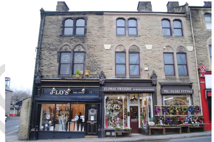
Figure 33 Shop fronts on Lower Burnley Road, demonstrating sympathetic design and original features.
