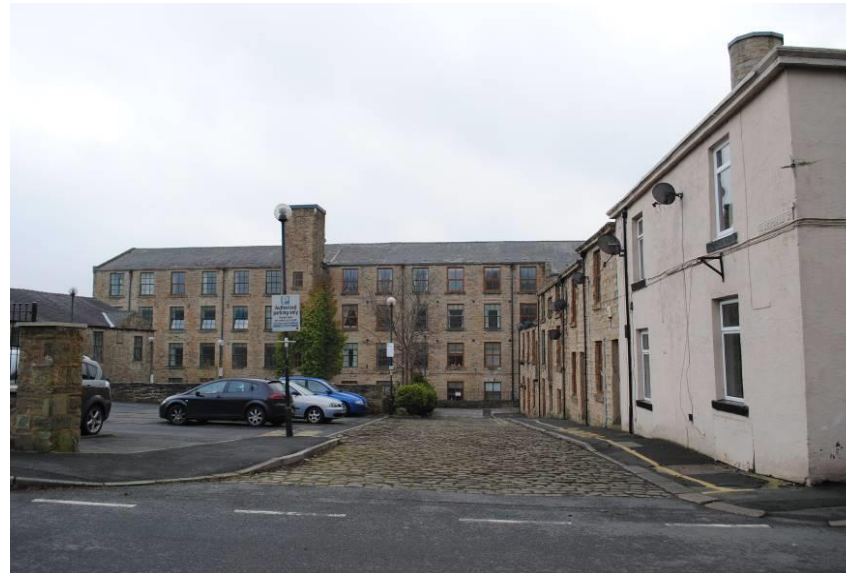
Figure 45 Victoria Mill from Guy Street
