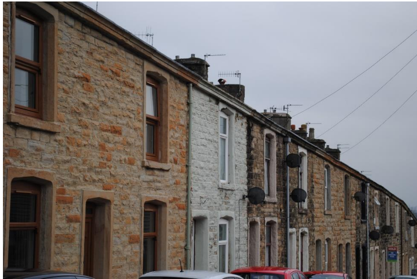
Figure 68 Satellite dishes on Alma Street
