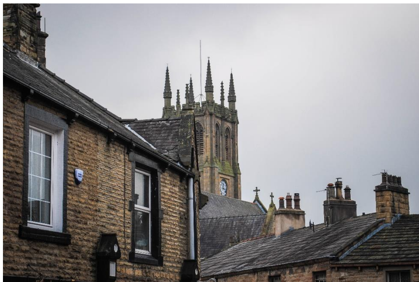
Figure 11 St Leonard's Tower peeking above the roofscape.
