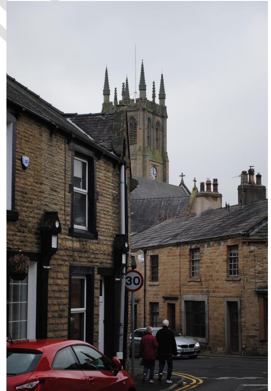
Figure 47 St Leonard's Church Tower from Guy Street
