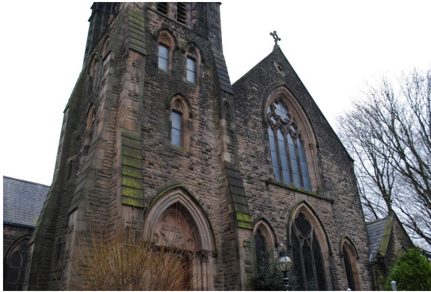
Figure 76 Unitarian Chapel from Church Street
